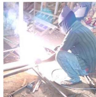
Figure 1. Workers Welding in a Squatting Position (Mindhayani, 2021)
